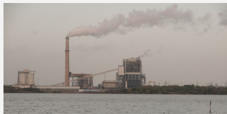
Gibbons Creek Generating Station
