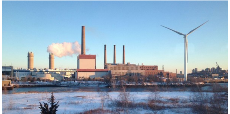
Mystic Generating Station, on the Mystic River in Everett, Massachusetts. A wind turbine owned by the local water authority to power a pumping station is on the right.
